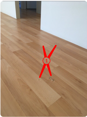
Image: 8 1: Damage and wear to wood-look flooring along left side of area
